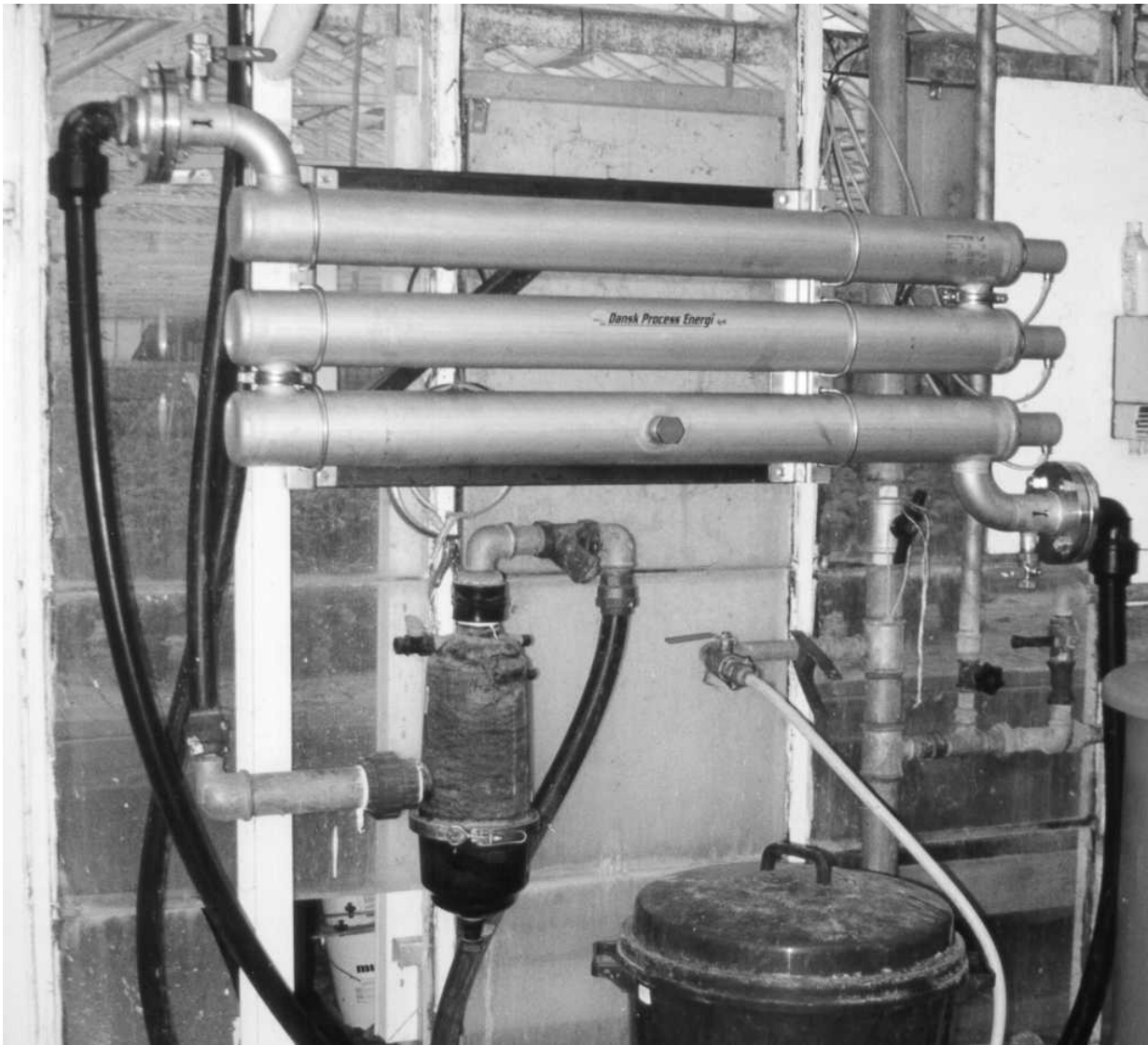
Figur 8: Testinstallation af AQS-UV LM3/200 SW
